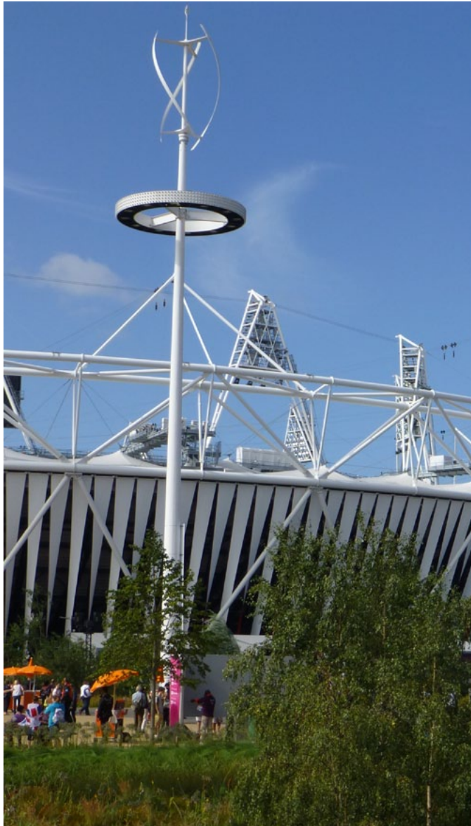
One of seven micro-wind turbines on the Olympic Park that provided a visible dimension to the low carbon Games, while the low embodied carbon of the materials used in venue construction achieved some of our biggest wins.
