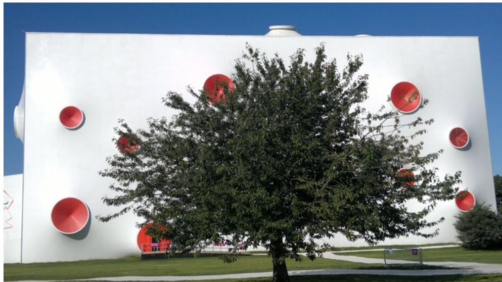
Temporary shooting venue at Royal Artillery Barracks - reducing the embodied impacts of construction materials was one of the priorities of our carbon management strategy
