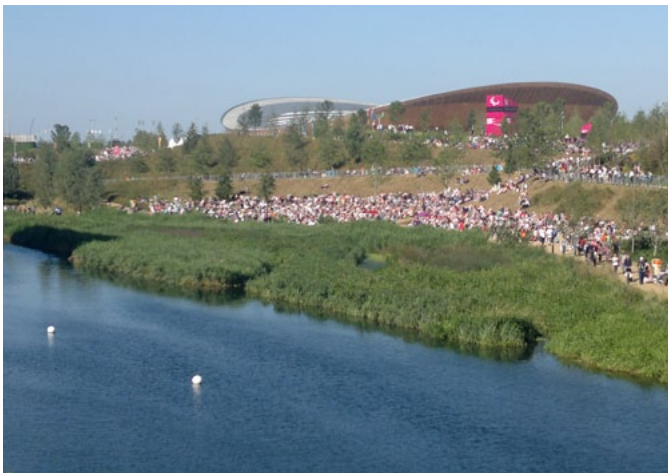
After (2012): new wetland bowl in the north of the Olympic Park during the Games. This area provides valuable new habitats, amenity and flood relief.
